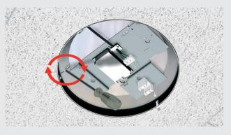
**3:** Push the shoe against the Troldtekt panel's upper edge and screw it tight. Install the electric cables.
