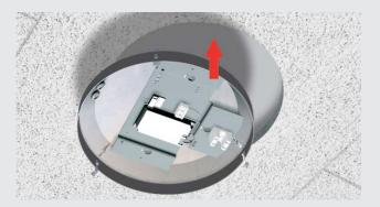
1: The Troldtekt panels are delivered with lamp cutouts. Place the armature in the lamp hole.
